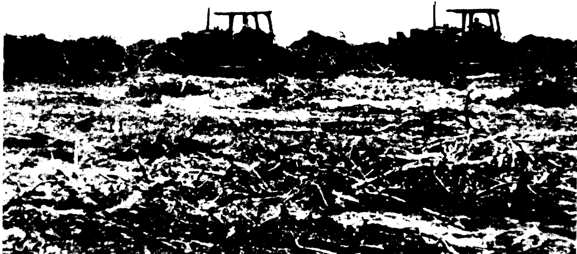
FIGURE 6-3. WINDROWING BRUSH ON ISLAND JANET. After brush was knocked down by the anchor chain, it was pushed into windrows. (July 1977)
