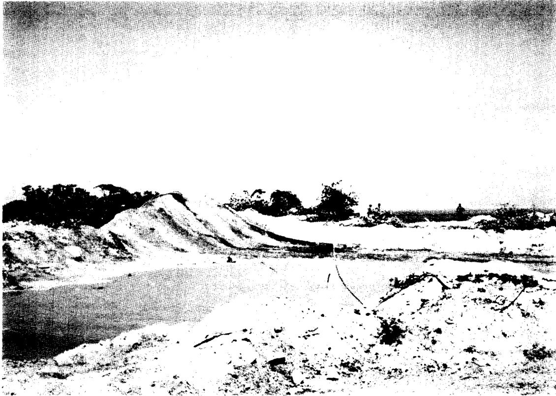
FIGURE 6-21. SUBSURFACE EXCISION ON ISLAND JANET. Soil was pushed out of the hole into a mound. The hole had standing water by the next day. Piled up soil was all removed, then the hole was backfilled and recontoured. (January 1979)
