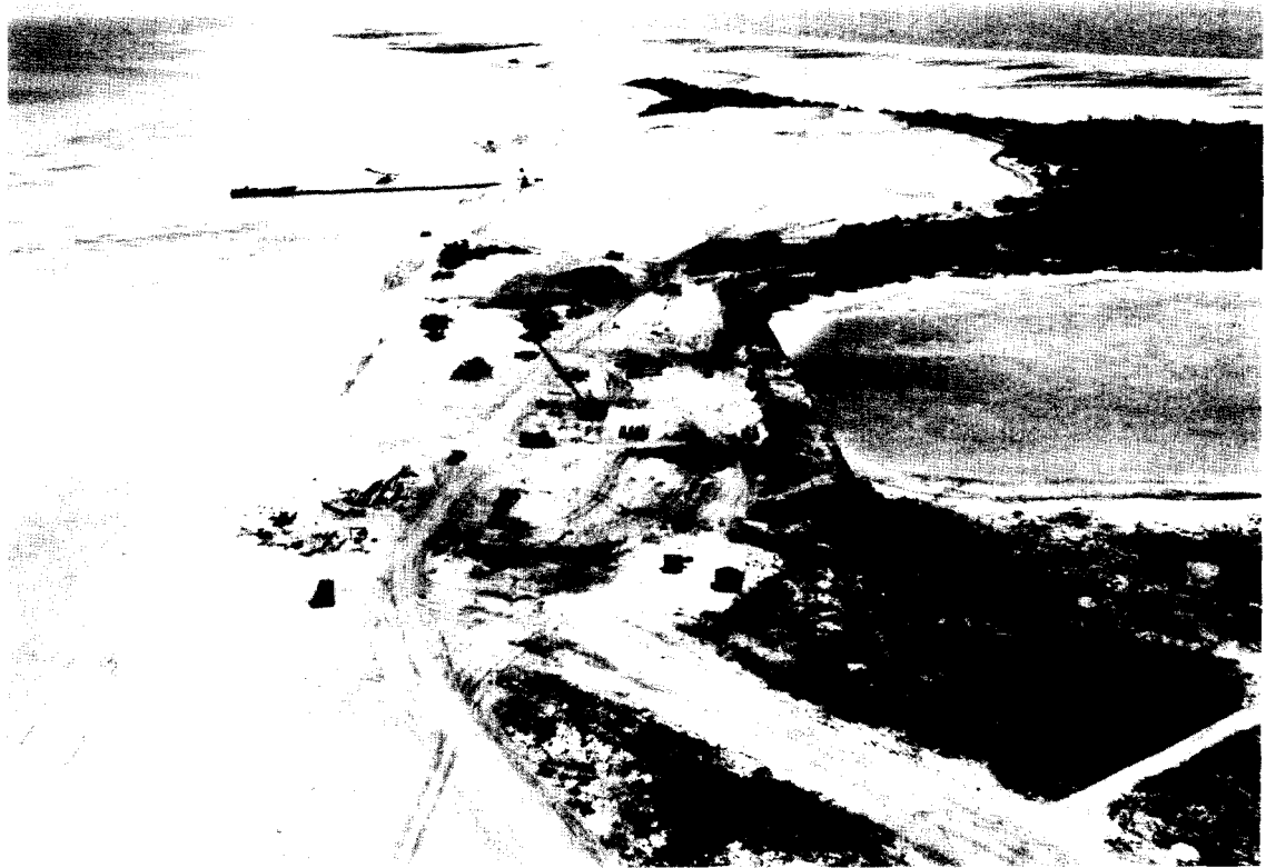
FIGURE 6-16. AOMON CRYPT AREA NEAR JOB COMPLETION. The last few sheetpile are being removed. Backfill material came from the beach in left foreground. The PACE area in the background has been totally recontoured. (June 1979)
