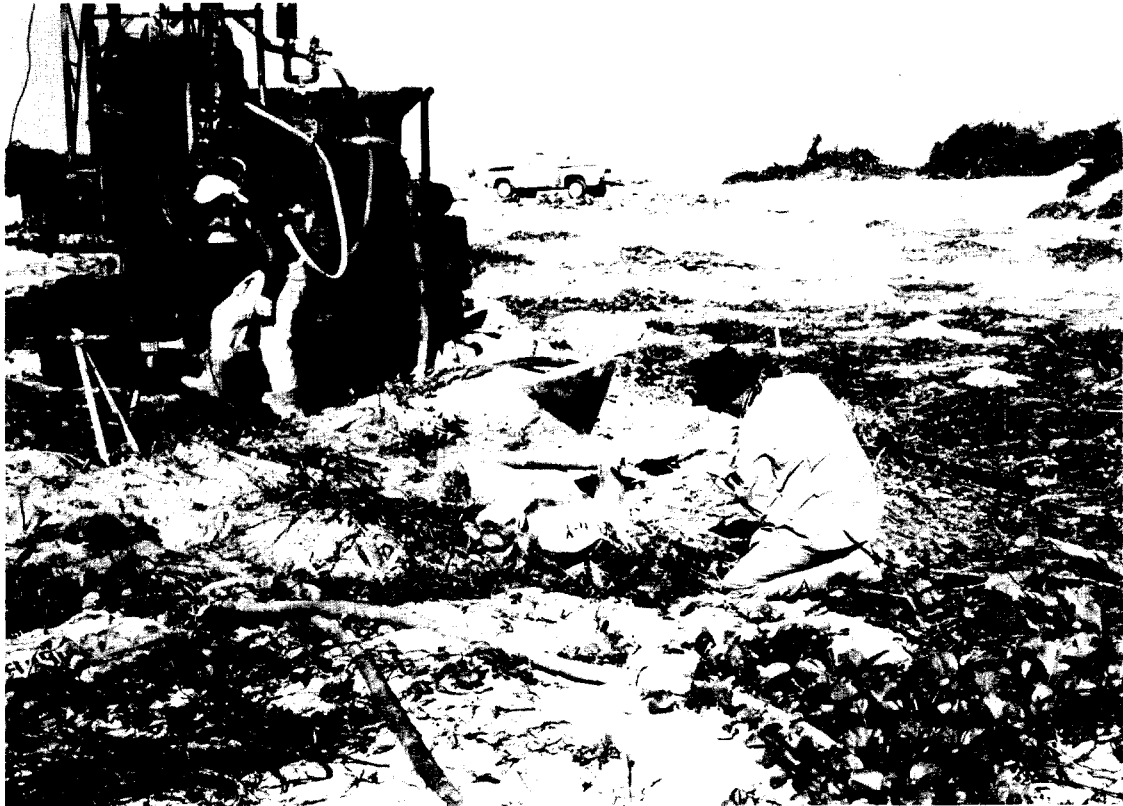
FIGURE 6-9. CORING DRILL AT THE AOMON CRYPT. The center monument area as viewed toward the west during drilling operations. (January 1979)
