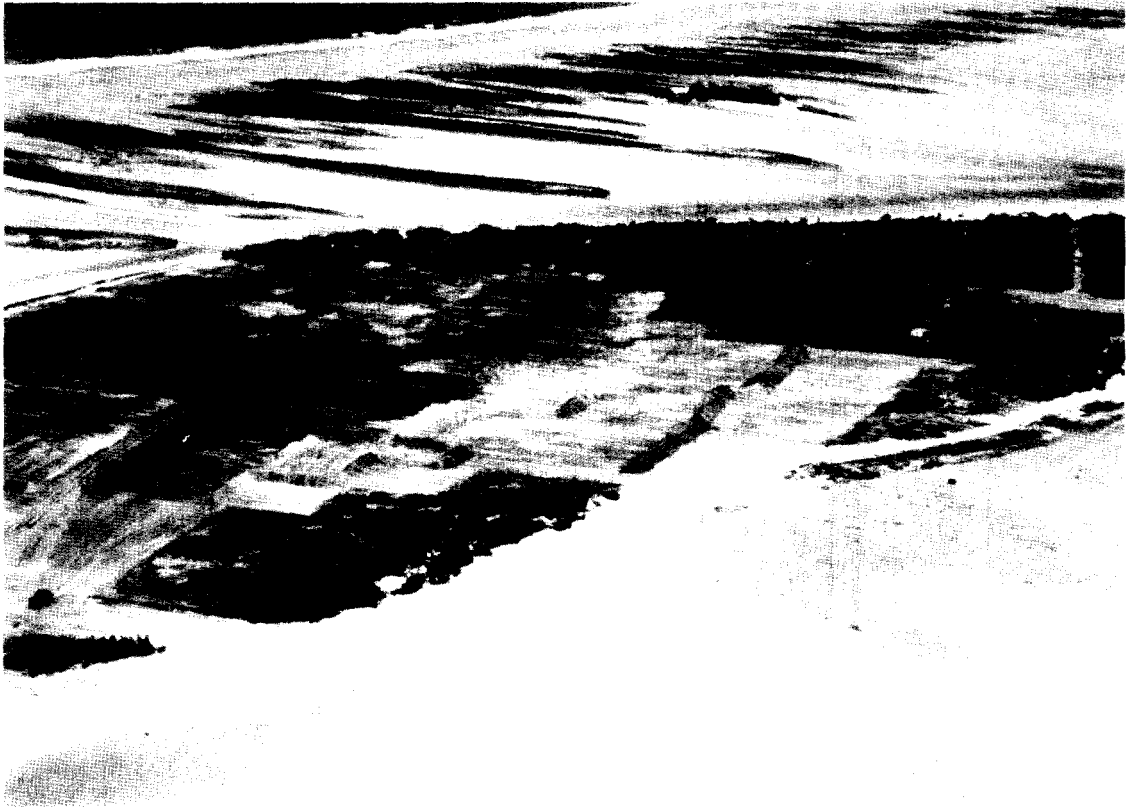
FIGURE 6-22. SURFACE SOIL REMOVAL FROM ISLAND PEARL. Soil was pushed into windrows, then hauled to a stockpile, at lower left, to await transport to Yvonne. Only a small area near right center required more than one soil "lift." View is almost due east. (June 1979)
