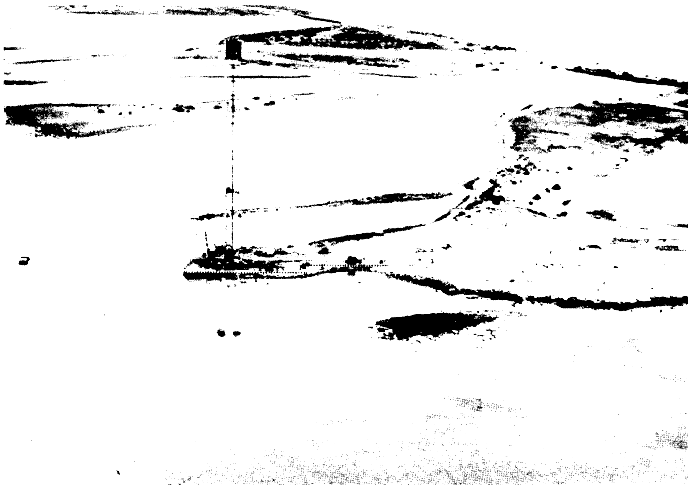
PLATE 9. ISLAND SALLY, NORTH TIP, SPRING, 1956. The tower for the KICKAPOO test was located on a jetty extension of the north tip of Sally. This positioning eliminated the need for dust suppression measures. Islands Tilda, Ursula and Vera are in the background.
