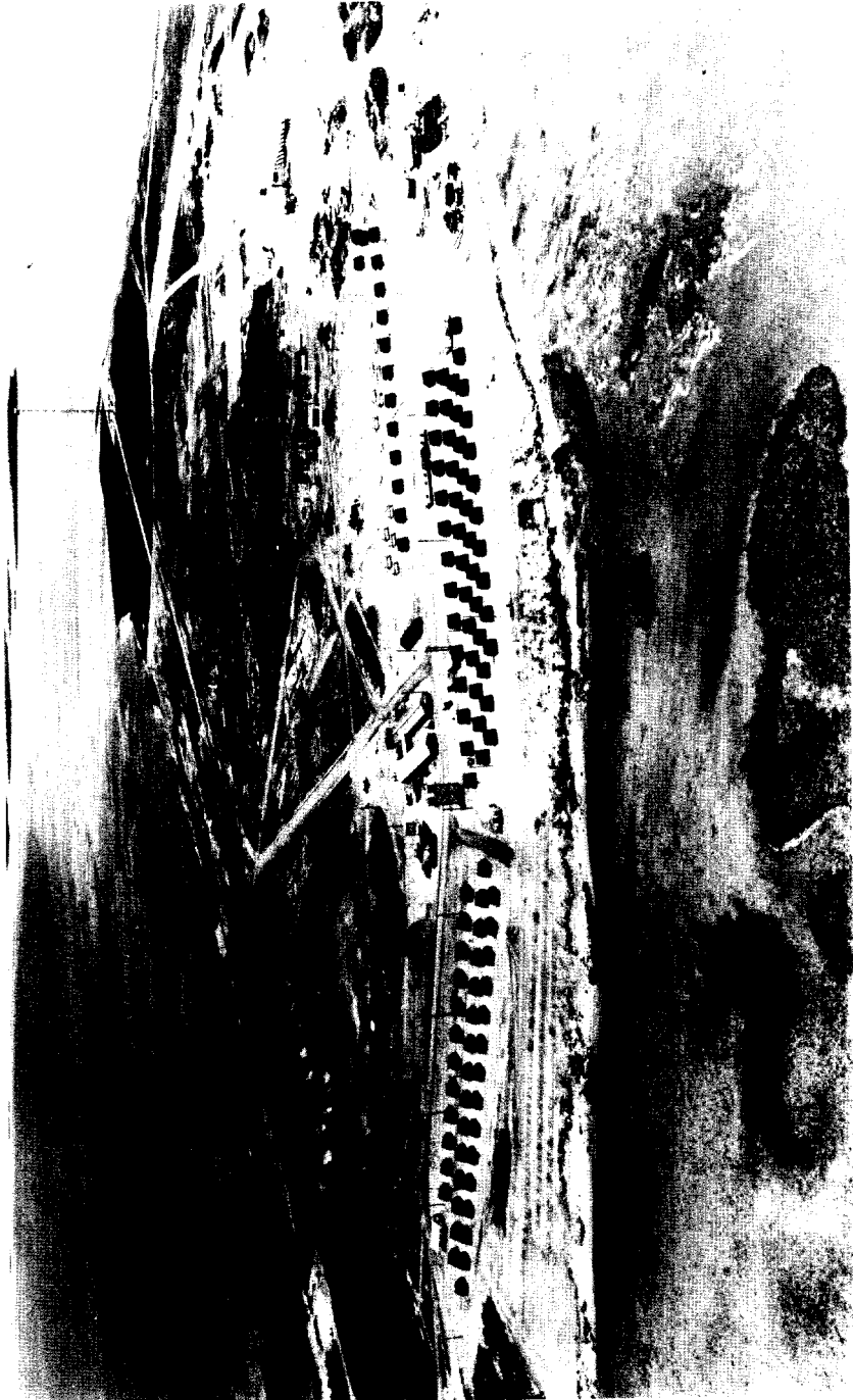
PLATE 5. ISLAND JANET, 10 JULY 1950. The tower and paving for the EASY test detonation are in position. Construction is in progress on the multistory test building, Station 3.1.1 (located toward the island center).
