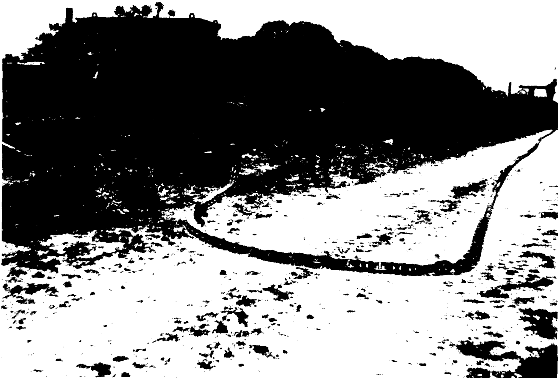
FIGURE 6-2. SYSTEM USED TO DEVEGETATE ISLAND JANET. The two bulldozers pulled the 200-foot anchor chain, stretched between them, across the brush. Vegetation was knocked down but not removed. (July 1977)
