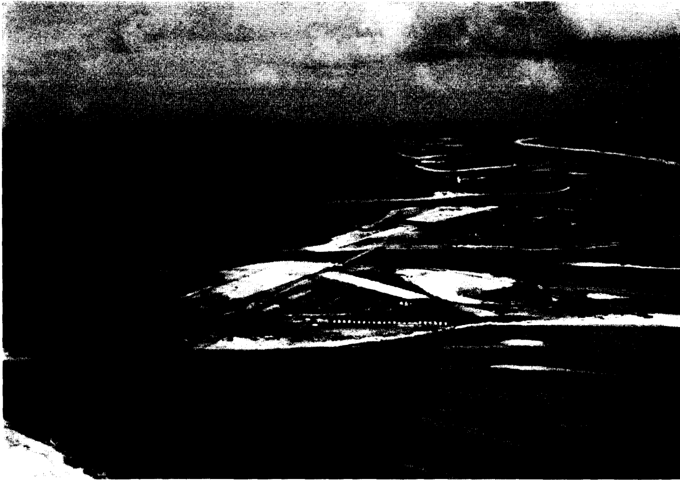
PLATE 8. ISLANDS TILDA AND SALLY, 30 MARCH 1948. Tilda is in the foreground, with Sally next, then Ruby, Pearl and Olive in the distance. The newly constructed sheetpile causeway, where the Aomon Crypt was later located, can be seen connecting Tilda with Sally. The tower for the YOKE test is located at the Ruby end of Sally.
