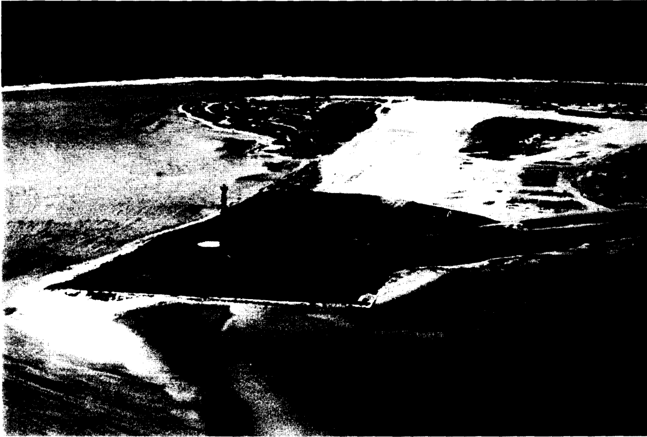
PLATE 4. ISLAND JANET, 30 MARCH 1948. Preparations for the 14 April X-RAY detonation included laying asphalt for dust suppression within a radius of 1000 feet of the test tower. The cleared area (the runway) is the only evidence that a fighter base existed here three years earlier.
